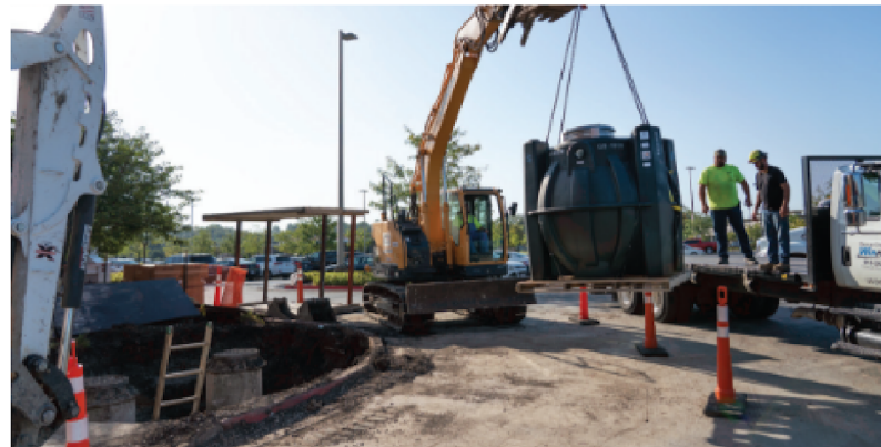
▲ Our new GB-1000 being installed at Costco in Independence, Missouri
